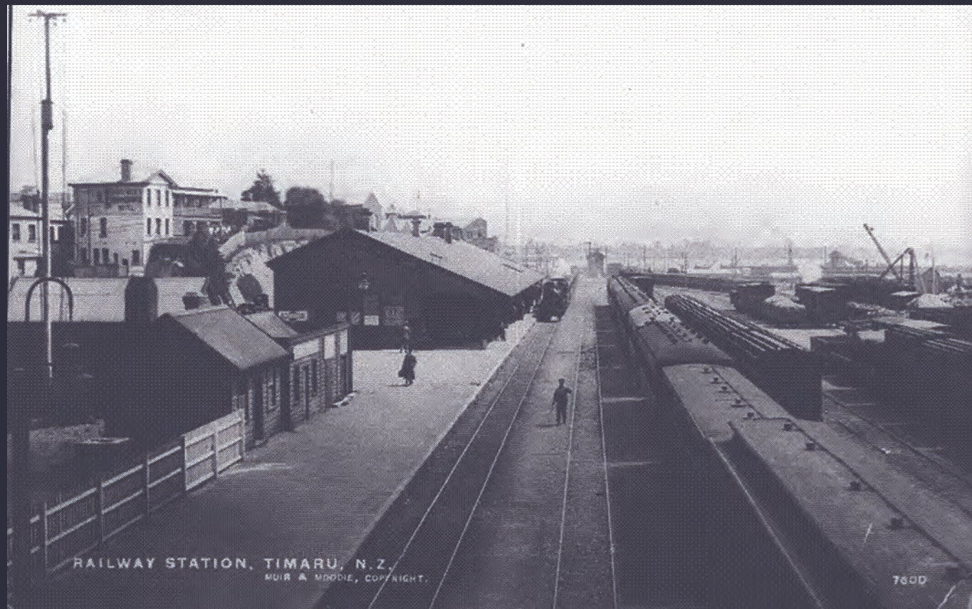
Timaru Railway Station.
