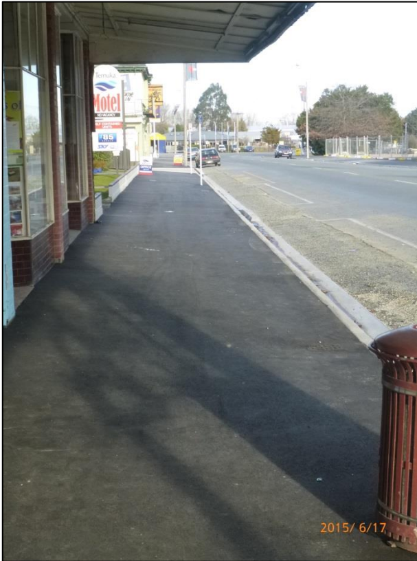
Figure 30 – New pavement south of Domain Avenue
