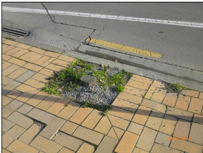
Figure 34 – Street tree removed - a new tree or the pavement have been reinstated
