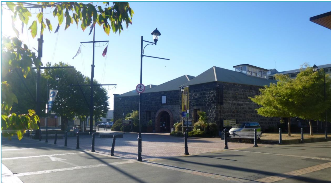
Figure 22 – Timaru’s Landing Services Building – Before (Top) and After Renovation (Bottom)
